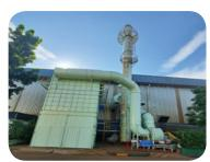
Installation of a wet scrubber system at ICP2 for the Shell Core process to enhance air treatment efficiency and improve workplace conditions by reducing chemical vapor and odor emissions.
