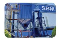
Installation of an additional dust collector system with a capacity of 1,000 CMM (increased from the original 570 CMM) at ICP2 for the Finishing & Grinding process, aimed at improving air pollution control efficiency.
