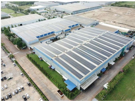
Figure 3 Picture of solar power installation of SBM Plant with an installed capacity of 1.5 MW
